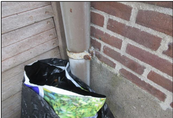
1. Roestvorming tpv gootbeugels: nazien/roestwerend behandelen, PM.
